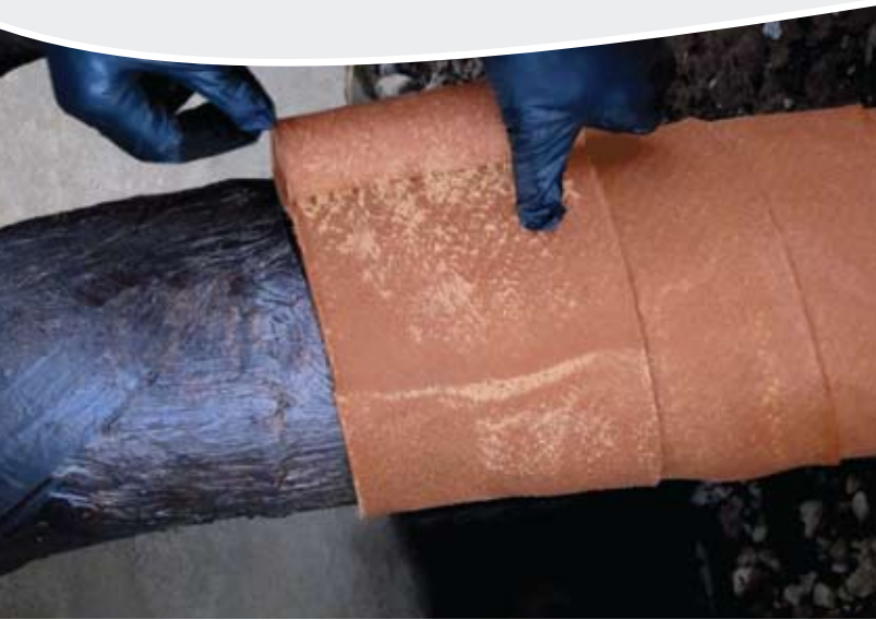
An easy-to-apply protection system for high-temperature applications, HT-3000 Wax-Tape requires minimal surface preparation.
